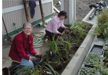
Bioretention during installation
