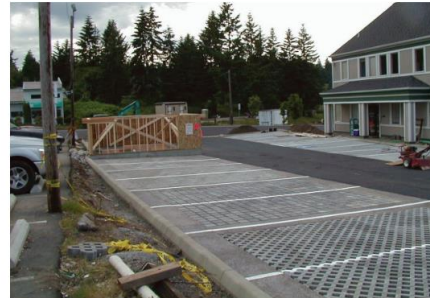
Permeable pavement installation
