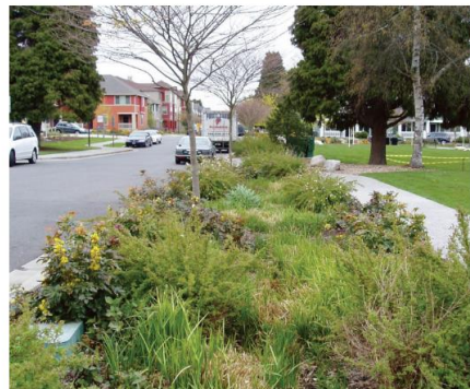
Established bioretention facility
